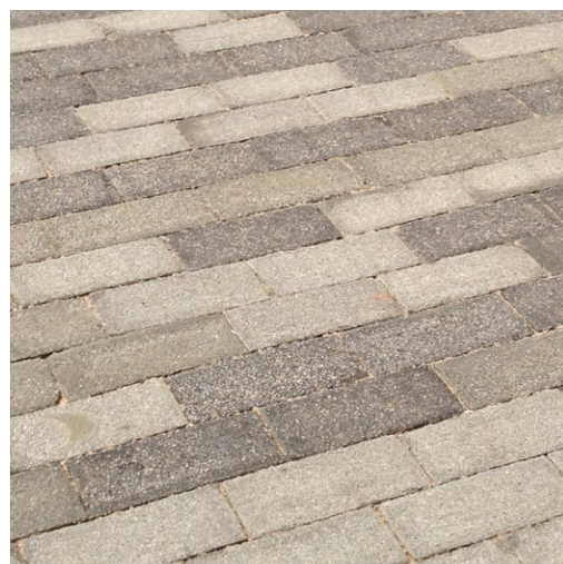
Vehicular Paving 1 Parking Bays UK Stone/Porphyry Size: 100mm width x 200mm length x minimum 75mm depth Alternative: High Quality Concrete Supplier: Hardscape
