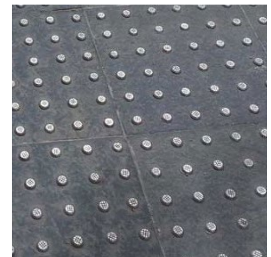
Tactiles: Metal tactile studs to formal crossing points
