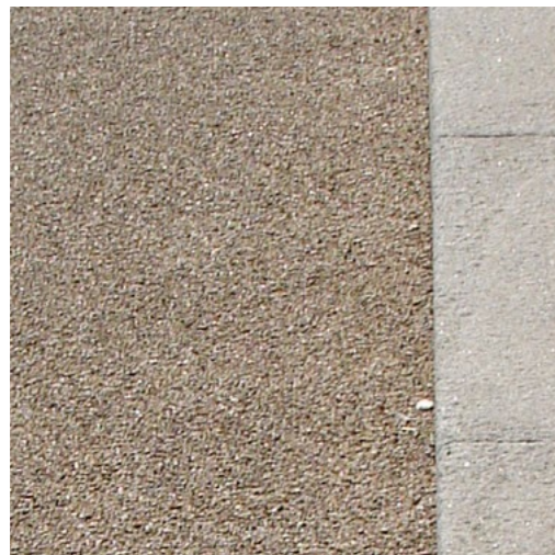
Pedestrian Paving 1 Pavements Resin Bound Gravel Product Ref. Addastone Size: 18mm surface depth Supplier: Addagrip Ltf
